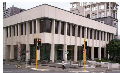
New Zealand's Court of Appeal building in Wellington, New Zealand
