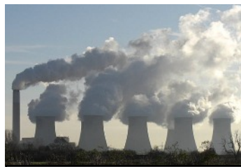
Ratcliffe-on-Soar Power Station in Nottinghamshire, England (Lady Wulfrun)
